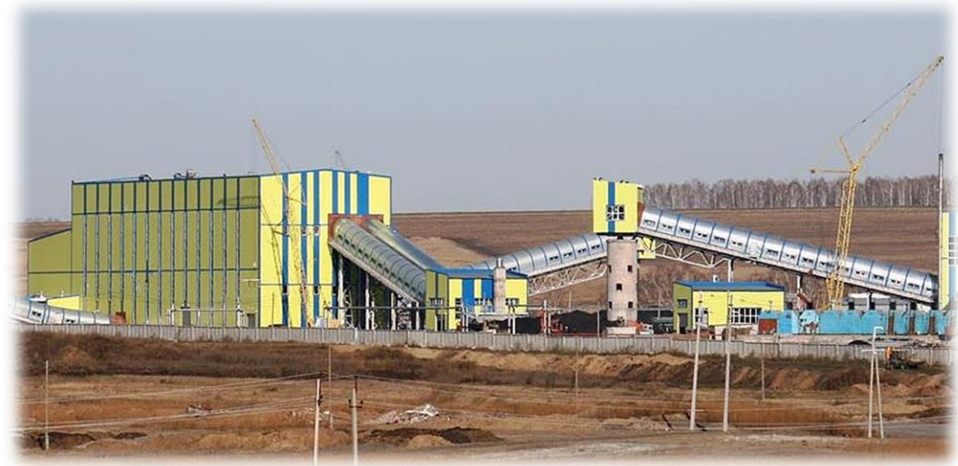
A modular CHPP example
