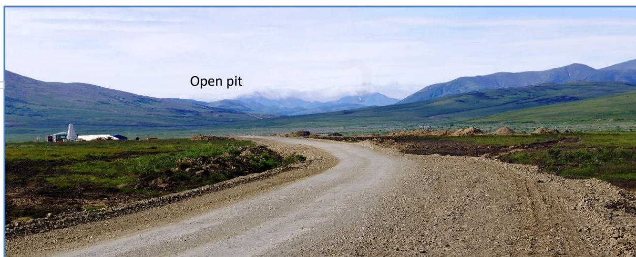
Project F haul road, the mine infrastructure area on the left and open pit in the distance
