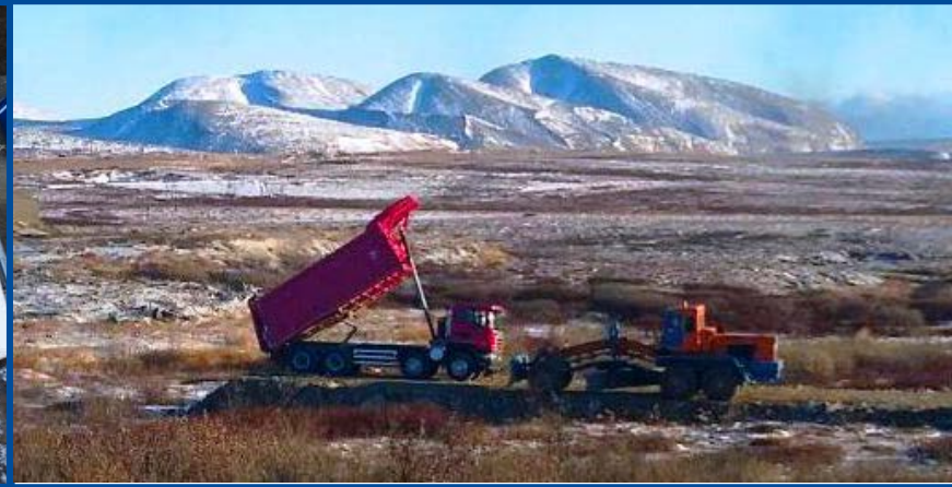
Road Construction – November 2016
