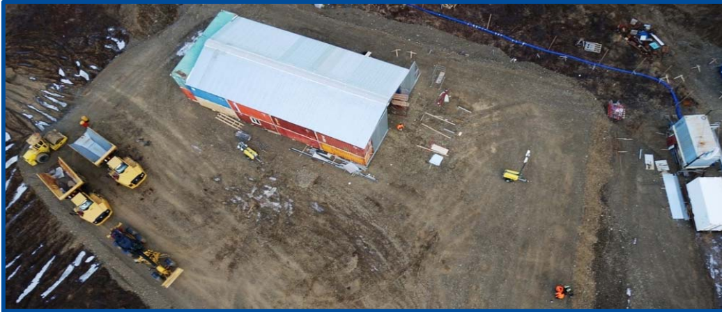
Infrastructure Construction – October 2016
