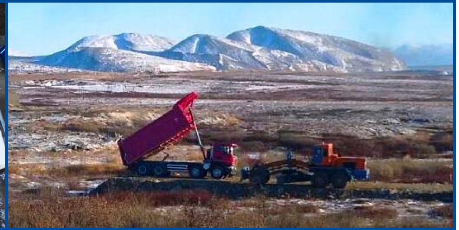
Road Construction – November 2016
