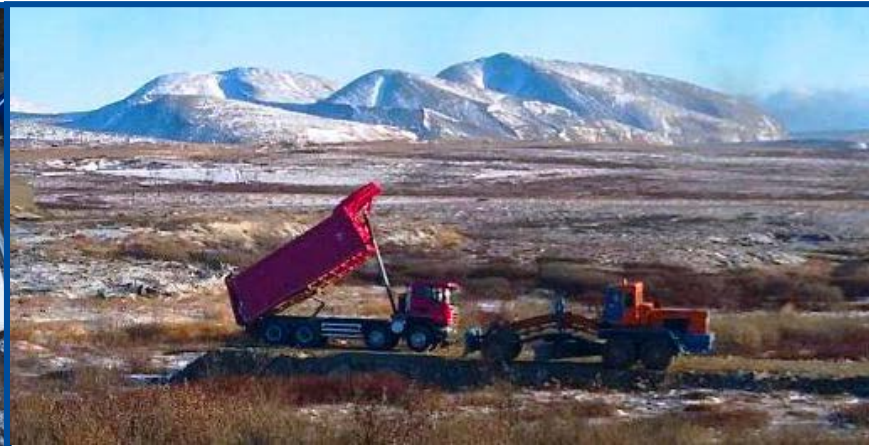
Road Construction – November 2016
