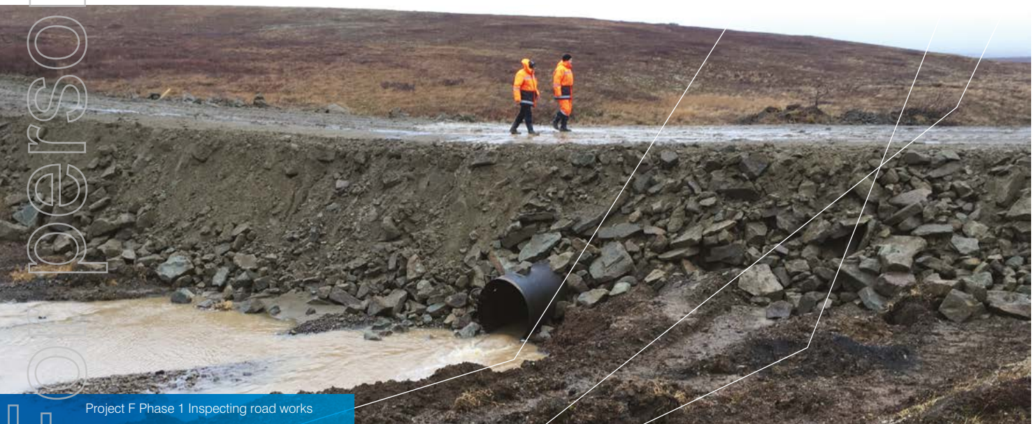
Project F Phase 1 Road construction works
