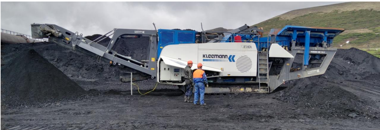
Commissioning the Kleemann Coal Crusher
