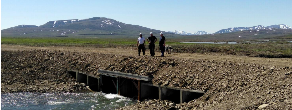
Completed section of road - Marcus Trost (Operations Manager), Anatoly Nikolaev (GM Operations) and Ivan Subbotin (Mining Manager) inspecting a completed river crossing.
