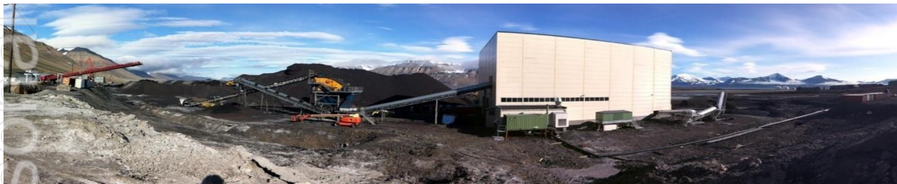
A modular CHPP example
