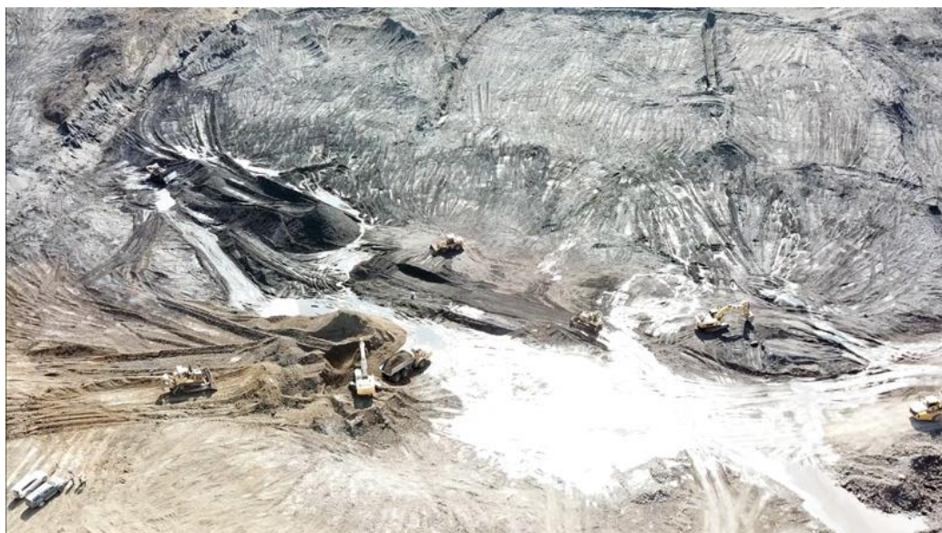
TIG Project F Pit operations summer 2018
